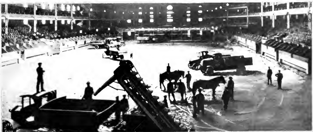
FIG. 26. ON MAY 3 AT 7:00 A.M. EXCAVATORS WITH HORSE DRAWN SCOOPS, PICKS, SHOVELS, LAZOS AND TRUCKS BEGAN TO CLEAR AWAY THE TANGARAK WHICH WAS LEFT FROM THE CIRCUS. AT 9:00 A.M. THE SHOT THE LINES, FOOT ELEVATIONS AND MADE THE SURVEY. THE DECORATIONS WERE STARTED (SEE "TRIPPE AROUND BOX FRONT" AND SOME OF THEM ARE IN PLACE. LAZOS) RIGHT OF PICTURE.
